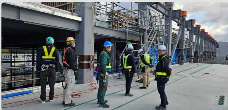
Regular safety inspections with project teams.
