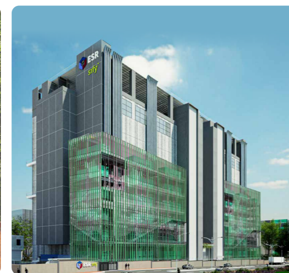
The new 60 MW ESR Rabale MU1 Data Centre has been pre-leased to a major information and communications technology company.
