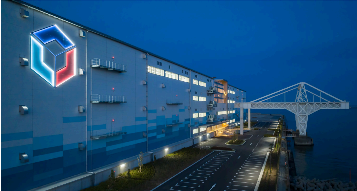
ESR Yokohama Sachiura Distribution Centre 2
